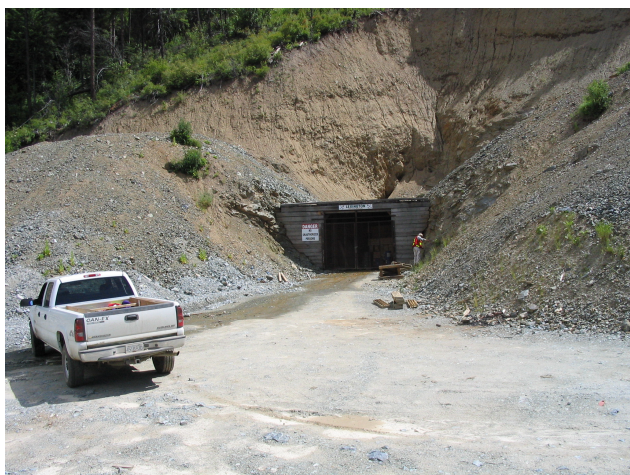
Figure 5.14. Grenoble portal on the Lexington property.
