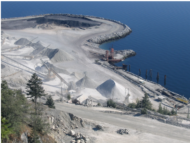
Figure 6.4. Gillies Bay quarry aggregate crushing plant and a stockpile of overseas bound coal from the Quinsam Coal mine.
