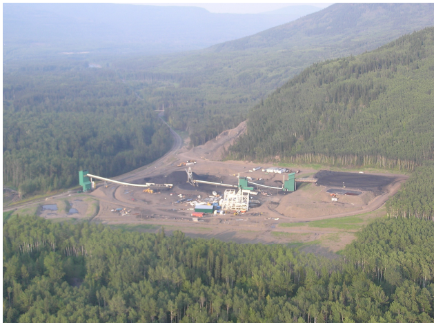
Figure 7.2. Willow Creek plant site and load-out facility.
