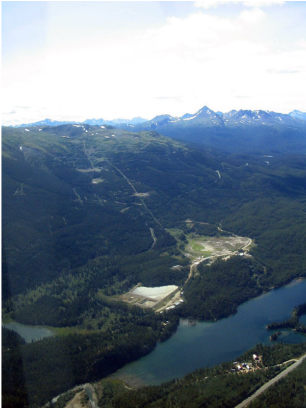
Photo 2. Looking easterly over the Table Mountain gold mine which re-opened in December, 2006 (photo courtesy of Cusac Gold Mines).
