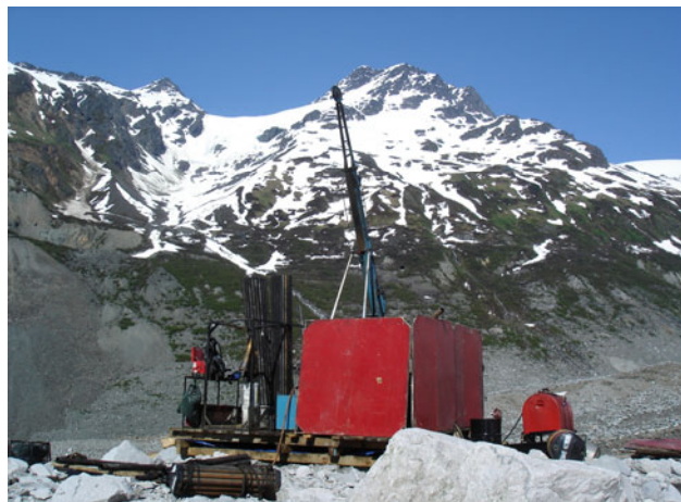
Figure 2.16. Drilling at Granduc, workings of the former copper mine underlie the mountain in the background.
