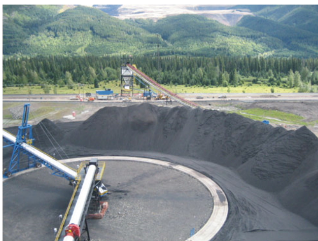
Figure 3.2. Stacker and rail loadout, Willow Creek mine.
