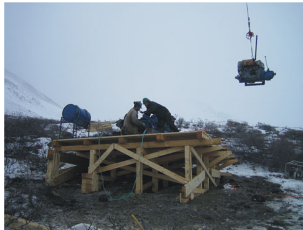
Figure 3.9. Erecting diamond drill on newly constructed pad, Trident property (photograph courtesy of Victor Koyanagi).
