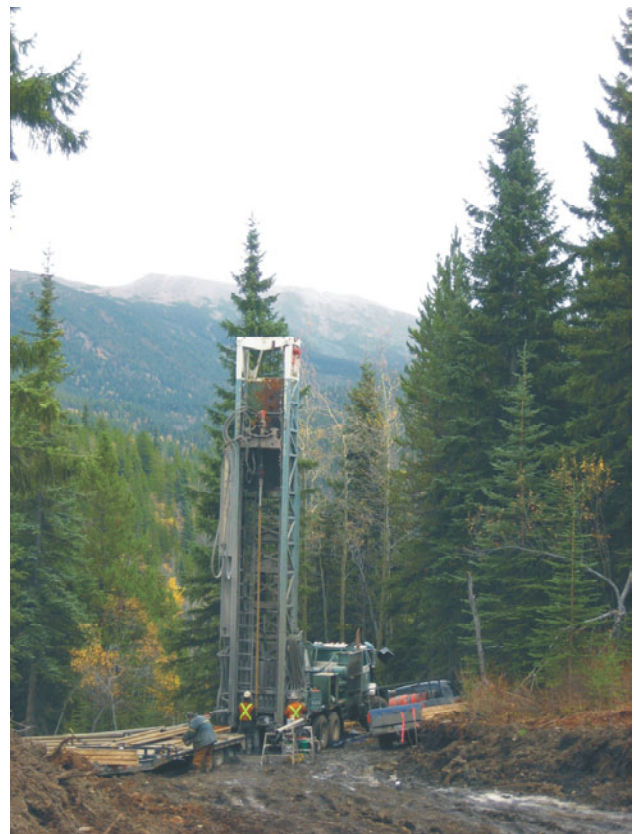
Figure 3.7. Air-rotary drilling to delineate coal resources, Horizon project.
