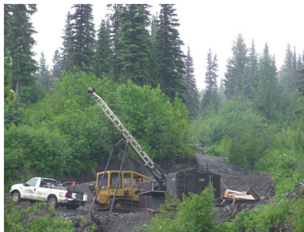
Figure 4.15. Drilling on the Spanish Mountain gold property.
