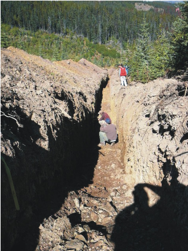
Figure 5.15. A trench across the JJ Zone at the Skoonka property.
