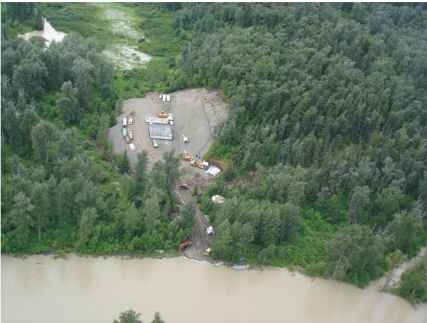
Figure 1.12. Construction camp near Big Bull, also the barge unloading point on a side channel of the Taku River.
