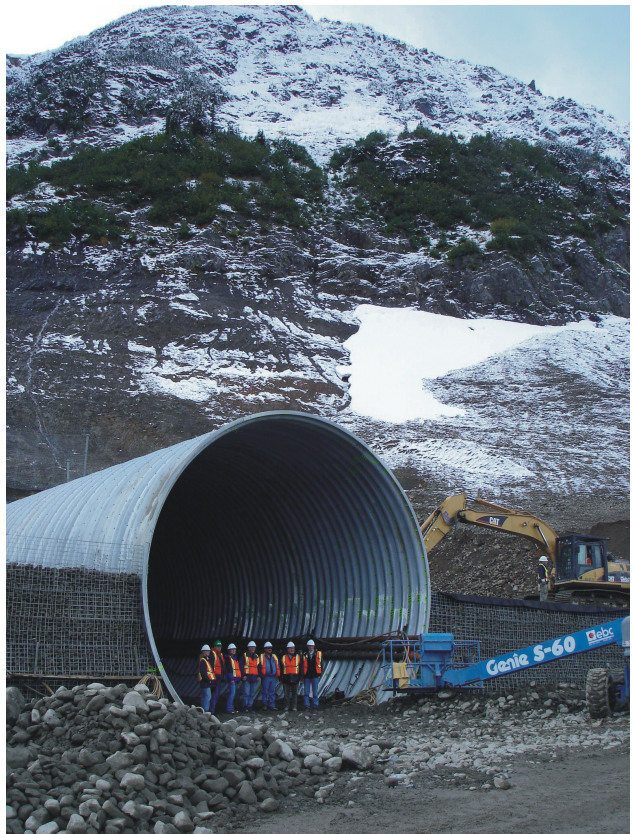
Figure 1.8. North portal of the Galore Creek access tunnel, entrance to the mine site in development.
