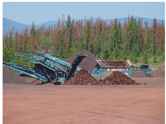
Figure 3.9. Screening operation at the Nazko quarry.
