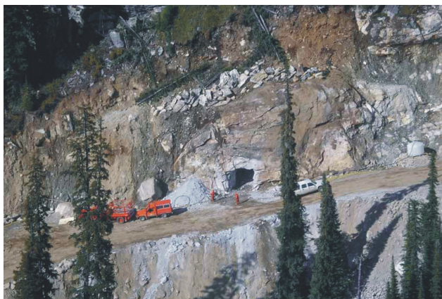
Figure 4.13. Portal to permit year round drilling of the E-Zone and Creek Zone at the Ruddock Creek property of Selkirk Metals Corp (Photo courtesy of Selkirk Metals Corp).
