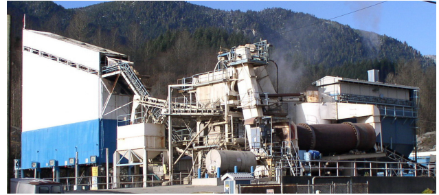
Figure 5.8. Jack Cewe's aggregate processing plant at Pipeline Road, Coquitlam.
