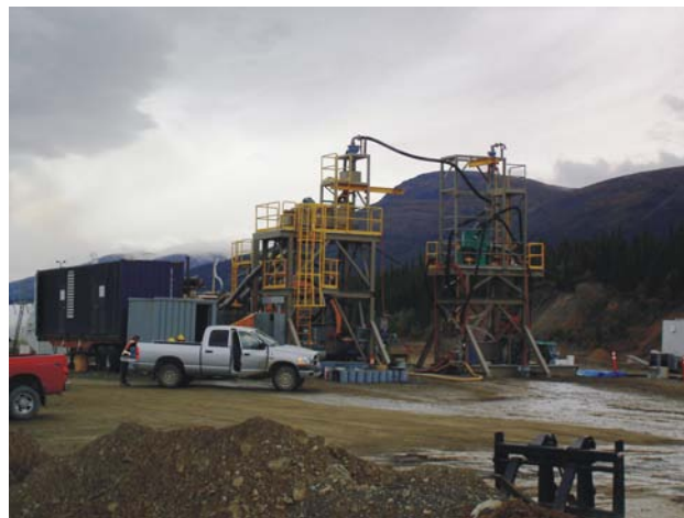
Figure 1.35. Pilot plant to recover gold on the Yellow Jacket (YJ) property.
