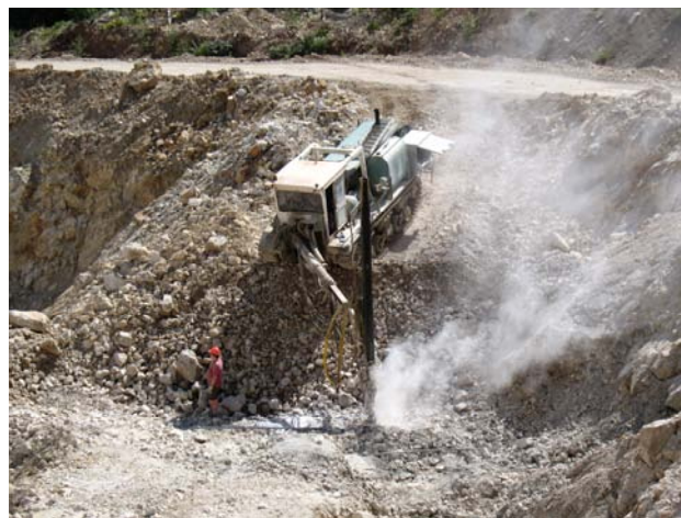
Figure 5.5. Drilling at Electra Gold’s Apple Bay quarry.
