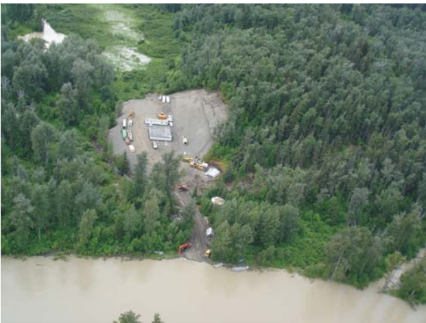
Figure 1.12. Construction camp near Big Bull, also the barge unloading point on a side channel of the Taku River.
