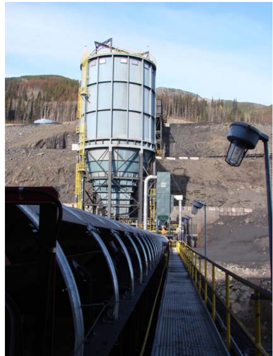
Figure 2.5. Wolverine Project: grizzly and conveyor at Perry Creek mine.
