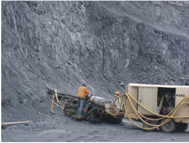
Figure 1.5. Drain holes are drilled in the highwall of the Main Zone Extension pit at Huckleberry mine.
