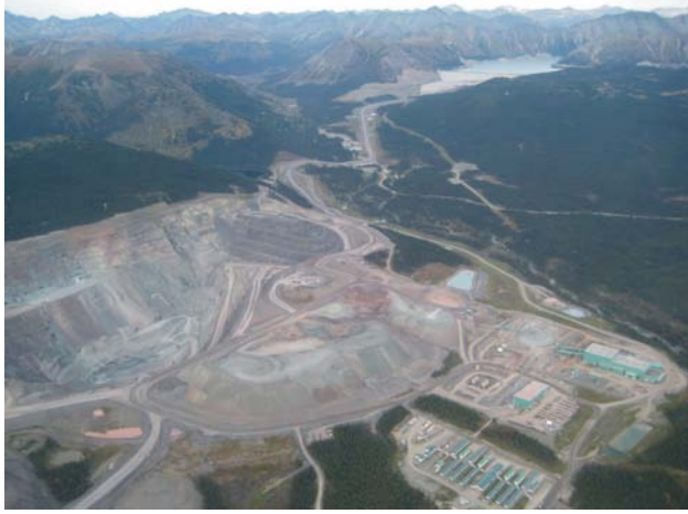
Figure 3.6. Crusher and Mill at the QR mine.
