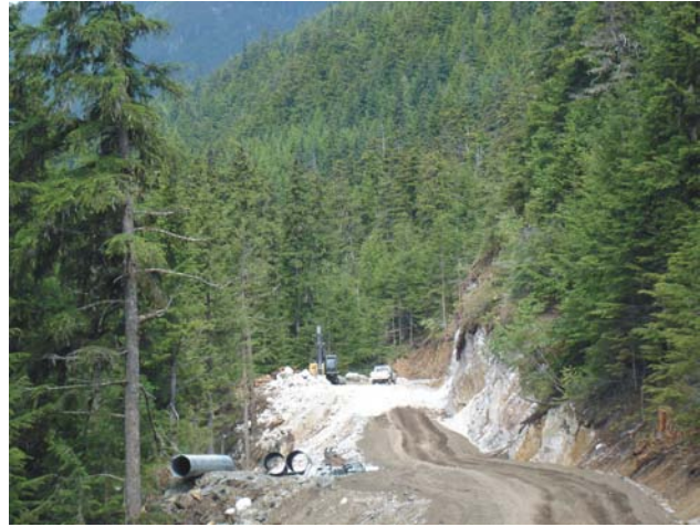
Figure 1.9. Tulsequah Chief Mine, new road will link the mine with a barge-landing site on the Taku River.
