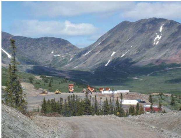
Figure 1.10. Ruby Creek, construction equipment parked on the new mine access road; tailings site in the distance.
