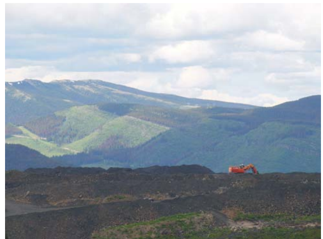
Figure 2.12. Site Preparation at Willow Creek North Zone.
