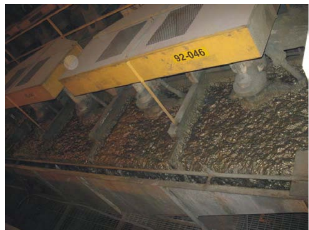
Figure 5.5. Flotation tanks at Breakwater Resource's Myra Falls Operations.
