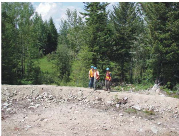
Figure 3.12. Drill pad reclamation at Gibraltar. (The barrier is to prevent runoff into the nearby wetland.)
