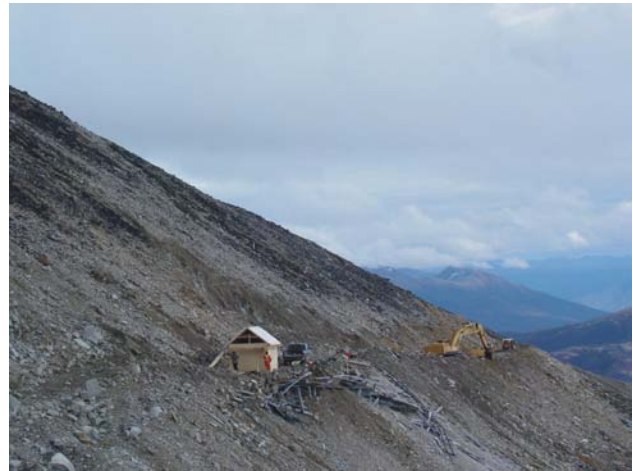
Figure 1.32. Cassiar Moly, access trail and exploration adit were re-opened.
