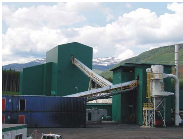
Figure 2.8. Grizzly, crusher and wash building at the Willow Creek mine site.
