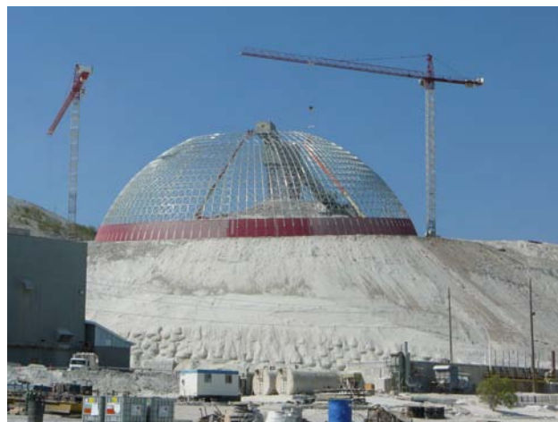
Figure 4.5. Geodesic domes over ore stockpiles being installed at the Highland Valley Copper mine near Logan Lake.
