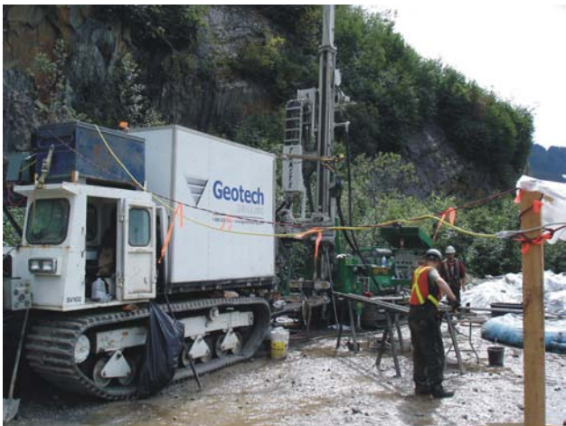
Figure 1.14. Kitsault, geotechnical drilling near the proposed plant site.
