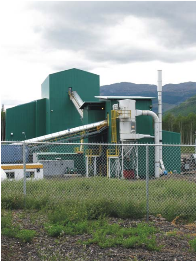
Figure 2.7. Willow Creek wash plant.
