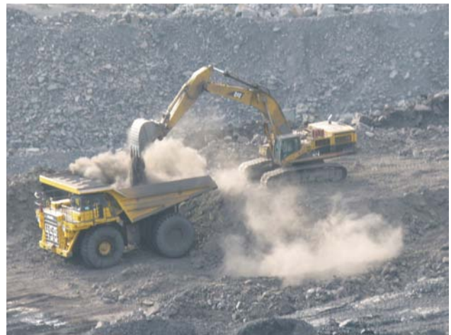
Figure 2.6. Moving waste rock at WCC's Wolverine Mine.
