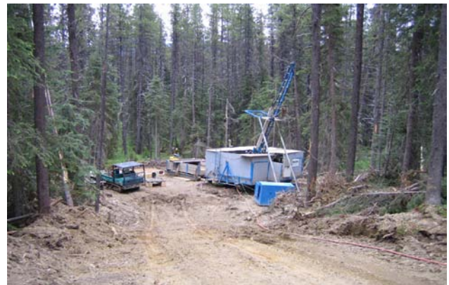
Figure 3.3. Kwanika; drilling on the copper-gold project.
