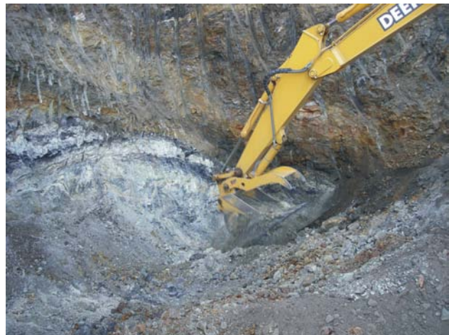
Figure 4.18b. Excavating the vein material at the Watson Bar property.
