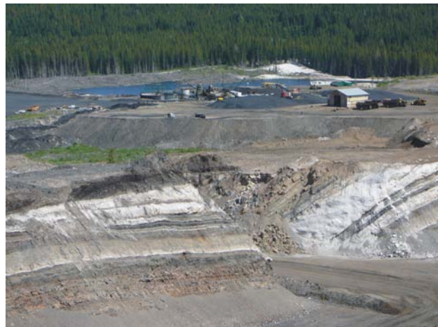
Figure 4.7. The idle Basin thermal coal mine near Coalmont was the subject of a feasibility study this year as part of a potential sale and resumption of mining.
