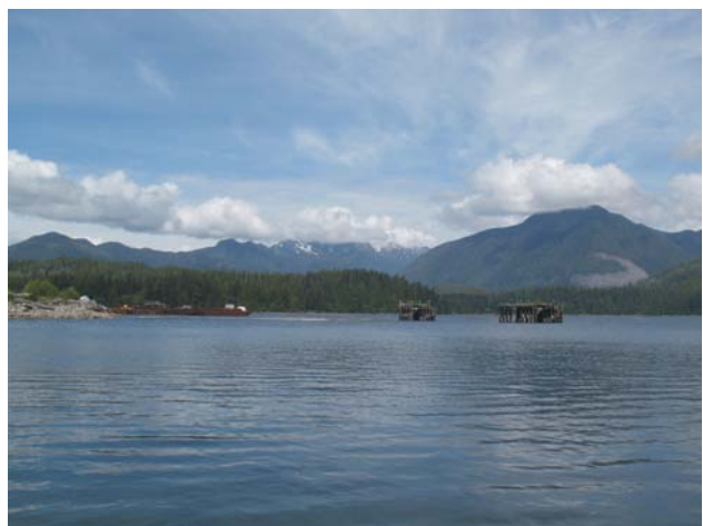
Figure 5.20. Pilings at the former Brynnor Mine's outloading facility in Toquart Inlet. Magnetite iron ore was shipped to Japanese steel mills from this site in the 1960's.
