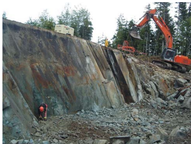
Figure 5.13. Haddington Island Quarry – photo courtesy of Haddington Island Stoneworks Ltd.
