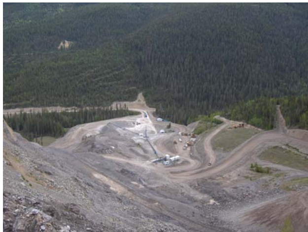
Figure 6.7. Handling and loadout facilities at the CertainTeed Gypsum Canada Elkhorn gypsum mine.
