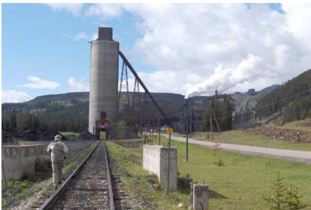
Figure 6.5. Rail loadout silo at Teck Coal Limited's Greenhills Operations. The coal preparation facilities are on the opposite side of the highway to the silo. The wash plant is on the sky line in the distance, and the dryer is immediately opposite the silo in the middle distance.
