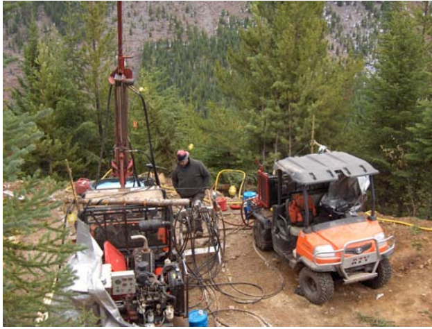
Figure 6.20. Diamond drilling on Spectrum Mining Corporation's Rock Canyon Creek project.
