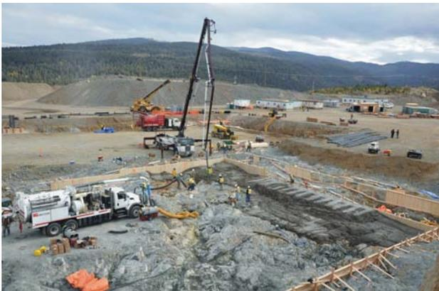
Figure 4.12. Foundations being poured this fall will allow the construction of a new mill building at the Copper Mountain mine development to begin in the spring of 2010 (photo courtesy of Copper Mountain Mining Corporation).
