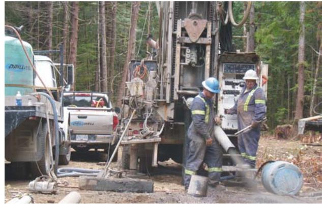
Figure 5.18. Driving in casing for a drill hole on the Raven coal project.
