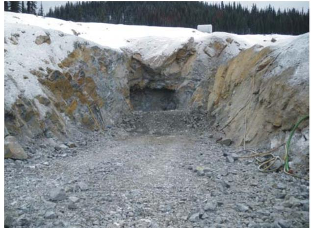
Figure 4.16. The start of a portal to exploit the Jewelry Box vein at the Bonaparte Gold property of Encore Renaissance Resources Corp north of Kamloops.
