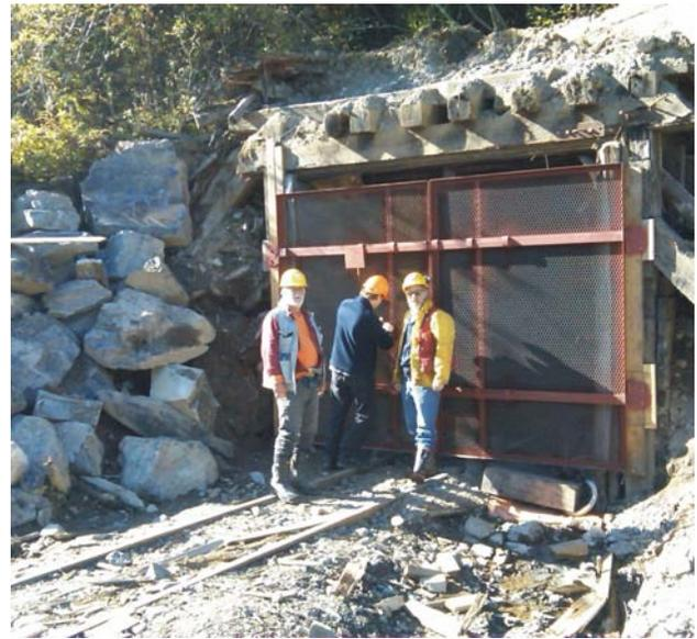
Figure 5.17. The portal at the former Carolin Mine was re-timbered as part of the underground rehabilitation at the Ladner project. Photo courtesy Module Resources Incorporated.
