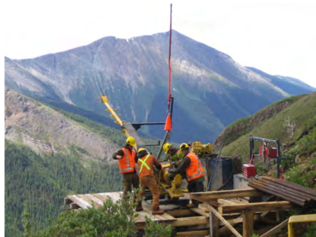
Figure 30. Drill move at Aley, image courtesy of Duncan McLeish.
