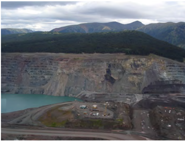
Figure 2. Kemess South mine showing failures on the north wall that result from graphite-bearing Asitka Group sedimentary rocks. A basement “high” of Takla rocks separates tailings in the West Pit from active mining in the East Pit.
