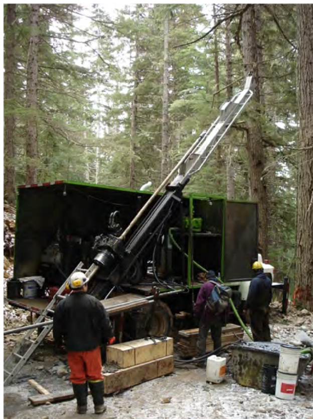
Figure 83. Truck-mounted diamond drill on the American Boy silver-gold project, north of Hazelton.
