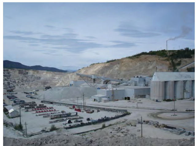
Figure 5. Endako molybdenum mine; mill, commissioned in 1965 continued in operation in June, 2010 while a new mill was under construction.
