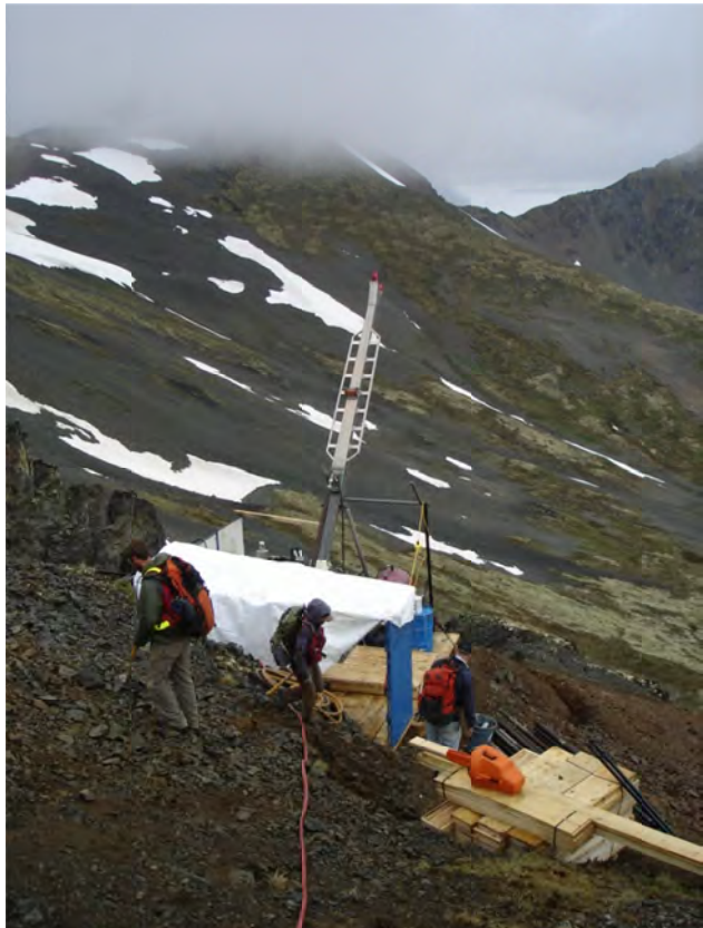
Figure 45. Drill set up on a ridge crest for the first hole on the GK (Glenora King) project to test below copper-gold showings on Winter Creek.
