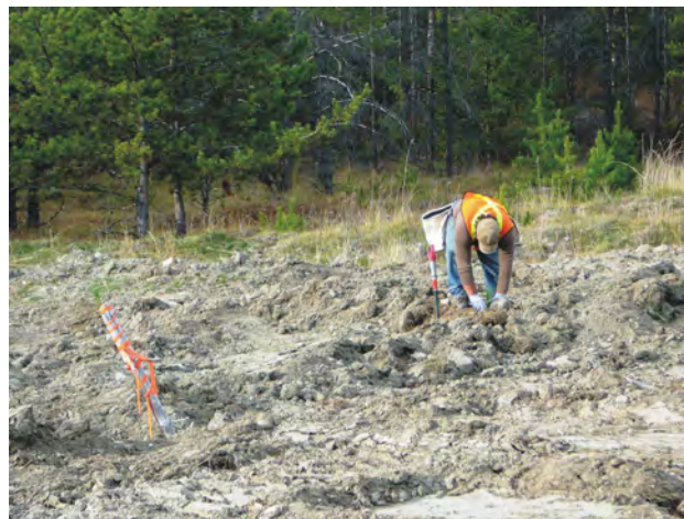
Figure 21. Ongoing reclamation of drill pads at the Woodjam project is an important undertaking for the operator, especially for such large programs that can go on for several years.
