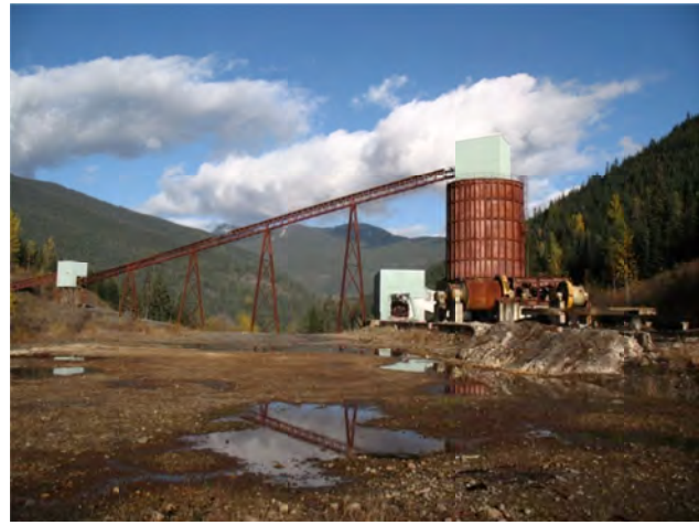
Figure 25. The Carolyn mine mill site at the Ladner gold project. The conveyor brought ore from an underground crusher.
