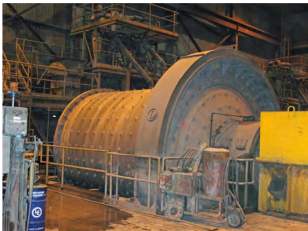
Figure 6. Mill improvements accounted for part of the capital expenditures at Myra Falls in 2010.
