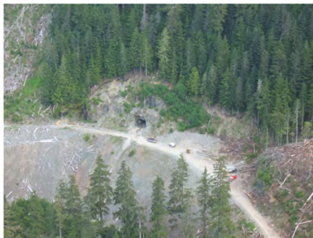
Figure 15. The portal of Westmin's 1989 exploration adit at Mineral Creek. It now houses a gravity mill used to process a bulk sample.
