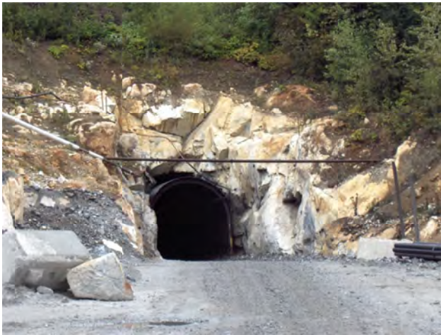
Figure 5. Adit #2 at Roca Mines Inc's MAX molybdenum mine near Trout Lake.
