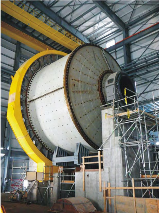
Figure 9. A partially installed 28 foot SAG mill at the New Afton gold-copper project near Kamloops awaits a mid-2012 start-up.
