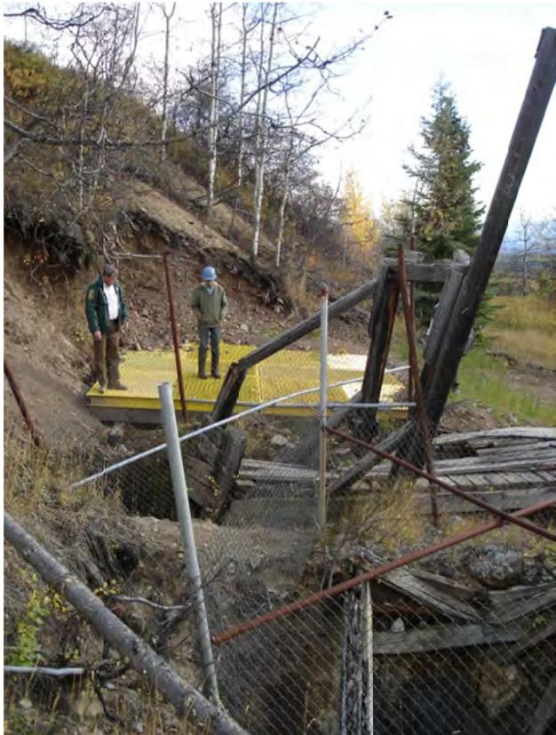
Figure 58. Silver Queen project; covers were installed on historic underground workings for safety reasons.
