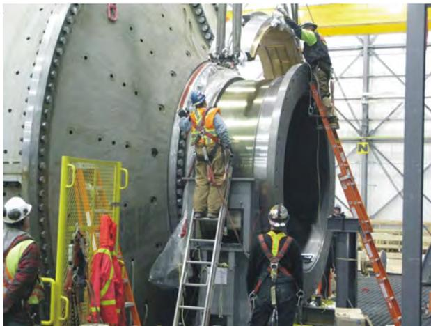
Figure 11c. Fitting a bearing on a mill (photo courtesy of Copper Mountain Mining Corporation).
