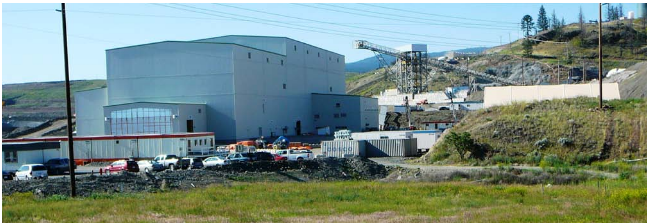
Figure 6. The ore conveyor emerges from the New Afton underground mine development scheduled for opening in 2012 after a five leg, 4.5 km long journey from preparatory underground mining operations.
