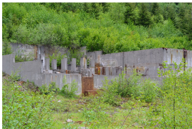
Figure 15. Mill foundations at the site of the past-producing Giant Mascot nickel-copper mine north of Hope. The mine operated mainly between 1958 and 1974. Exploration for nickel-copper-platinum group targets resumed on several neighbouring properties in 2011. Geoscience work on Giant Mascot is part of the federal Targeted Geoscience Initiative 4, involving GSC, BCGS and university partners.
