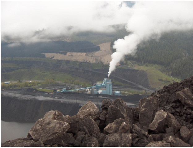
Figure 8. Coal preparation facilities at Coal Mountain (Teck Coal Limited).
