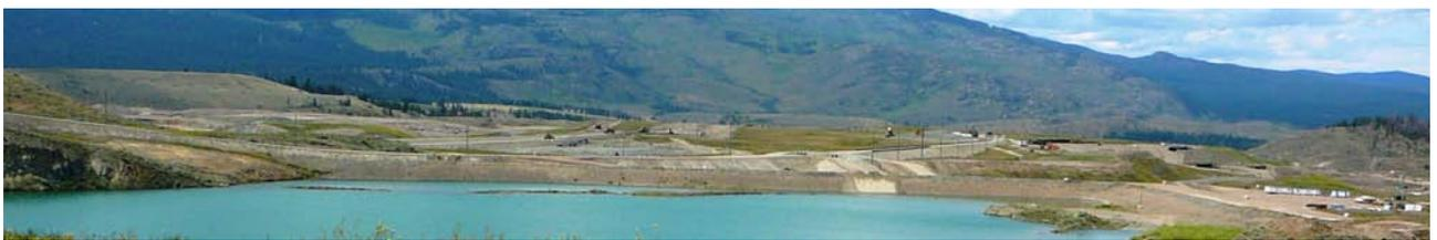
Figure 7. Site work is well underway at the New Afton project where a new tailings storage facility is being constructed and the Afton pit is being dewatered into the former Pothook pit.
