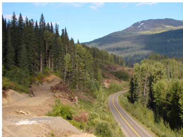
Figure 2.10. Northwest Transmission Line right-of-way clearing and pole foundation near Bell 2.
