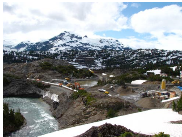
Figure 2.35. Big Missouri and Dilworth projects in the background of the Long Lake Hydro project headworks.
