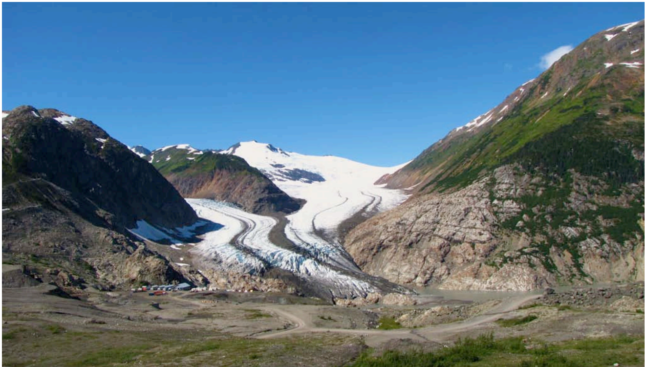
Figure 2.17. Looking west-northwest over the former Granduc mill site towards the Berendon Glacier. This is the portal entrance to the refurbished 17 km Tide Lake Tunnel which serviced the underground mine workings during past operation from 1970 - 1984.
