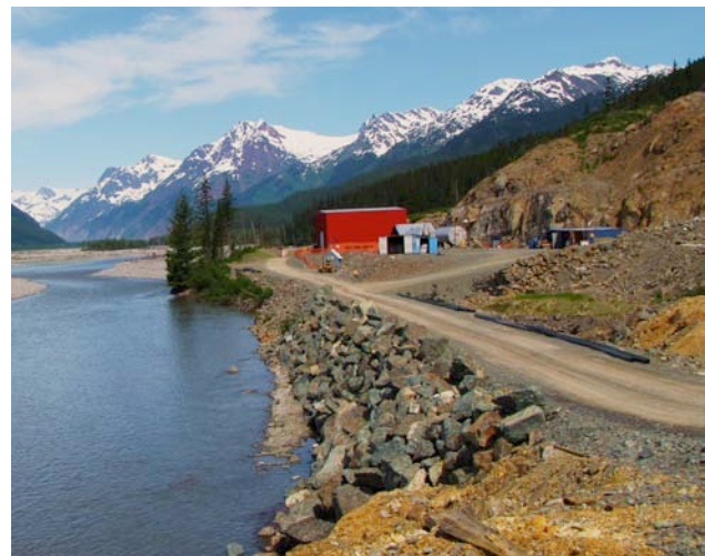
Figure 2.15. The water treatment plant at Tulsequah Chief reduced metal loading by 98%.
