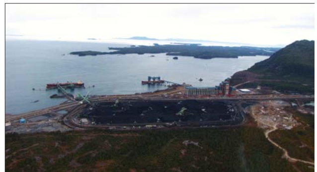
Figure 2.8. Expansion of the Ridley Island coal terminal is underway and receives fill material from nearby industrial quarries.
