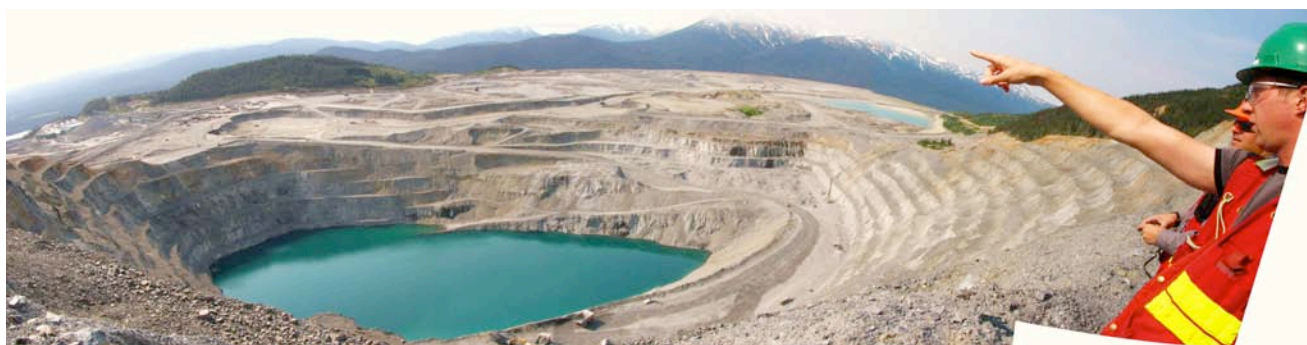
Figure 2.5. Overview of the Huckleberry Mine site looking southwest. Huckleberry Mines geologist Justin Schroff points out site components. Mill site is far left, stripping activities for the Main Zone Optimization are mid-left of center, active mining in the Main Zone Extension Pit is bottom center and mid-right of center.
