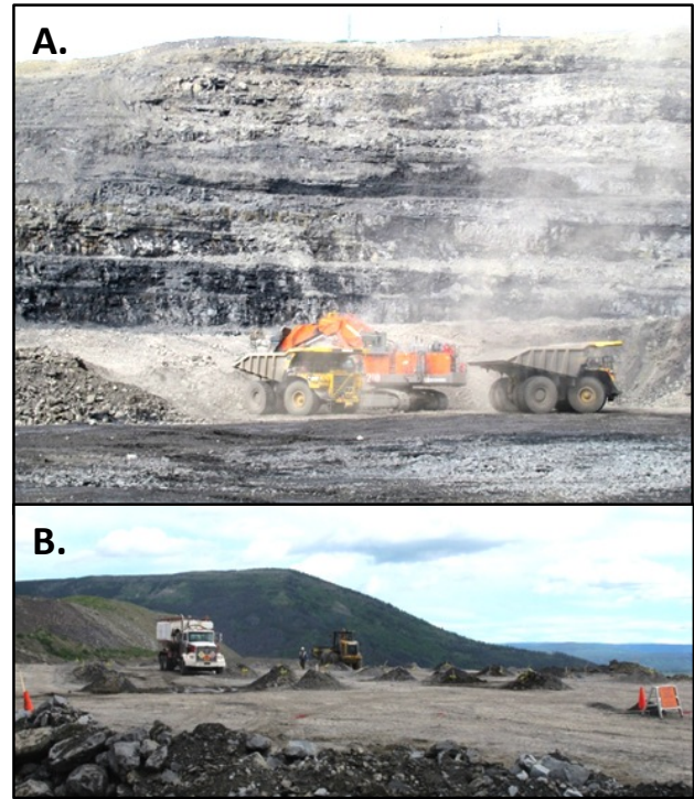
Figure 3.6. Perry Creek Mine – A. Digging to access G-seam in Phase 3B; B. Preparing to blast in Phase 4A.
