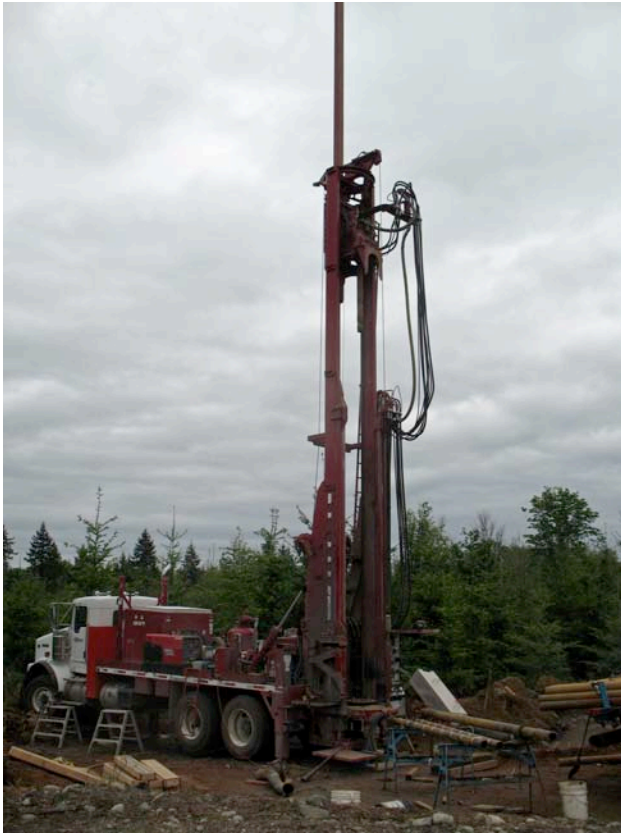
Figure 5.8. Rig preparing for drill move at Quinsam East.
