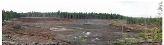
Figure 5.7. Site preparation of the 7 South area at Quinsam. A coal seam is exposed in the centre of the frame.
