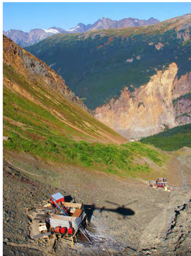
Figure 13. Directional deep drilling at the KSM project Deep Kerr zone with Sulphurets zone in the background. Photo credit Mike Savell, Seabridge Gold.
