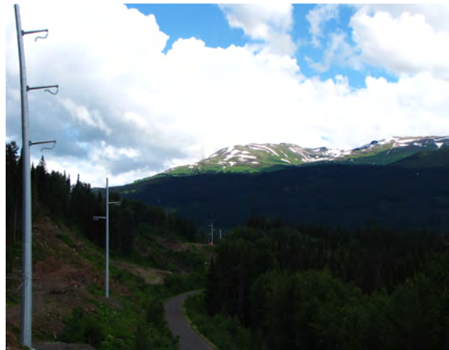
Figure 11. Northwest Transmission Line tower installation along Highway 37 near Bell 2.
