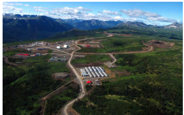
Figure 10. Mine construction at Imperial Metals Red Chris.
