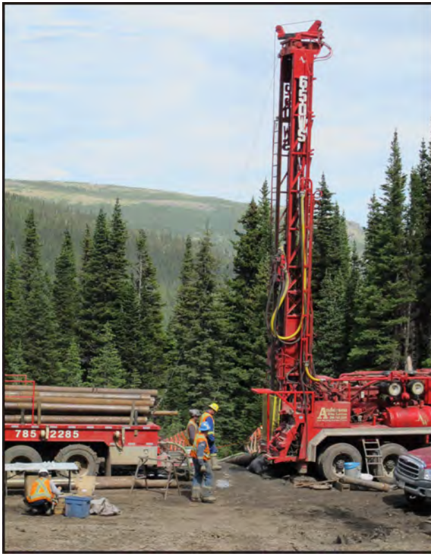
Figure 16. Roman Northwest – View north at LDC drilling.
