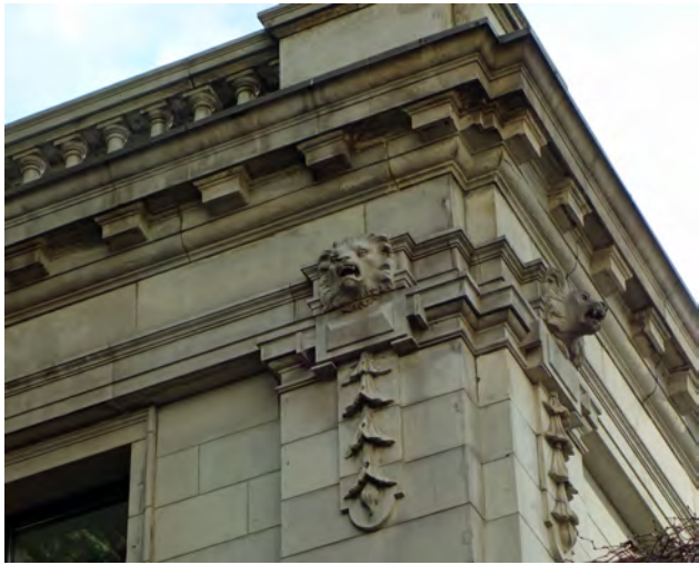
Figure 10. Haddington Island Andesite is found on historic buildings and monuments in Vancouver and Victoria. These are details on the Vancouver Art Gallery, constructed as the Provincial Court House in 1906-1912. The quarry on Haddington Island re-opened in 2004 and supplies material for restorations as well as new buildings and monuments.
