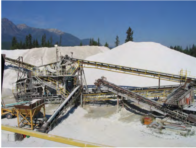
Figure 11. Silica sand at the Moberley mine (Heemskirk Canada Ltd). The mine currently produces a variety of silica products, and is currently evaluating facility expansion plans to supply frac sand to the oil and gas industry. Frac sand is used as a proppant for wellbore stimulation. Photo by Dave Grieve.
