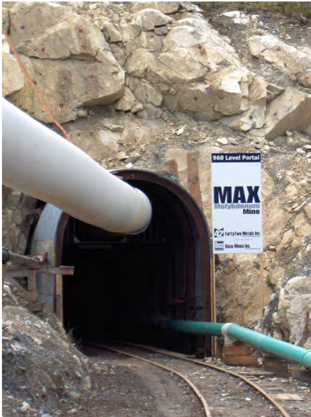
Figure 20. Entrance to 960-level portal at the MAX mine. Production at the molybdenum mine was suspended in 2010 after sill pillar stability issues. Operation resumed in 2011, but was later suspended again due to commodity prices. In 2013, Discovery Ventures Inc was granted conditional approval to acquire all issued and outstanding shares of FortyTwo Metals Inc, a subsidiary of Roca Mines. FortyTwo holds assets, including the MAX Mine and associated crushing, milling and concentrating facilities, tailings storage facilities, mineral claims, mining leases, and other licences and holdings. Photo taken by Dave Grieve.
