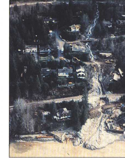
The Vancouver to Squamish highway has been affected by 14 major debris torrents since 1906. Twelve lives have been lost and 11 bridges, 4 homes and numerous structures have been damaged or destroyed. Not one of these 14 slide events was larger than 20 000 cubic metres (photo courtesy of the Ministry of Transportation and Highways).
