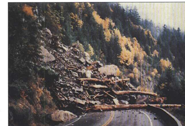
In 1991, a rock slide near Loggers Creek closed the Sea-to-Sky Highway for 12 days and cost $7 million for repairs and preventative structures (photo courtesy of the Ministry of Transportation and Highways).
