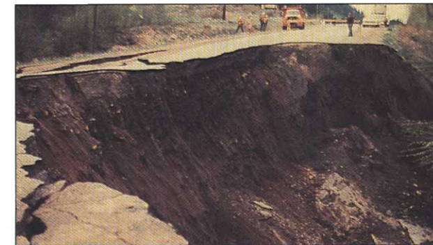
The Thuya Creek landslide near Little Fort occurred in 1972 and removed much of the roadway (photo courtesy of the Ministry of Transportation and Highways).
