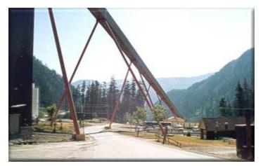
Boliden Westimin's Myra Falls Operations Conveyor belt housing from HW mine to mill.
