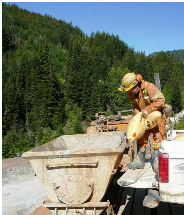
Figure 32. Loading explosives into an ore cart at the Bralorne mine.
