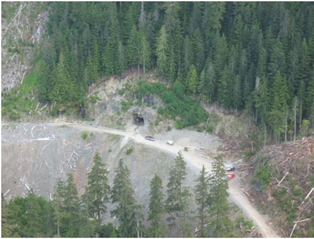
Figure 39. The portal of Westmin's 1989 exploration adit at Mineral Creek. It now houses a gravity mill used to process a bulk sample.
