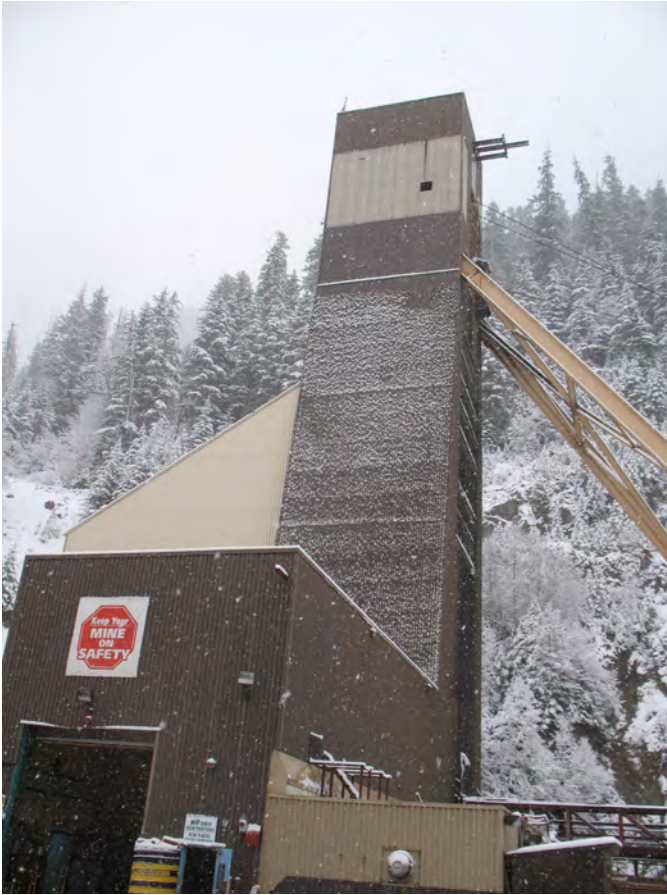
Fig. 7. The HW headframe at Myra Falls, an underground Zn-Cu-Pb-Ag-Au producer on Vancouver Island. Exploration is ongoing at this Kuroko-type VMS camp.
