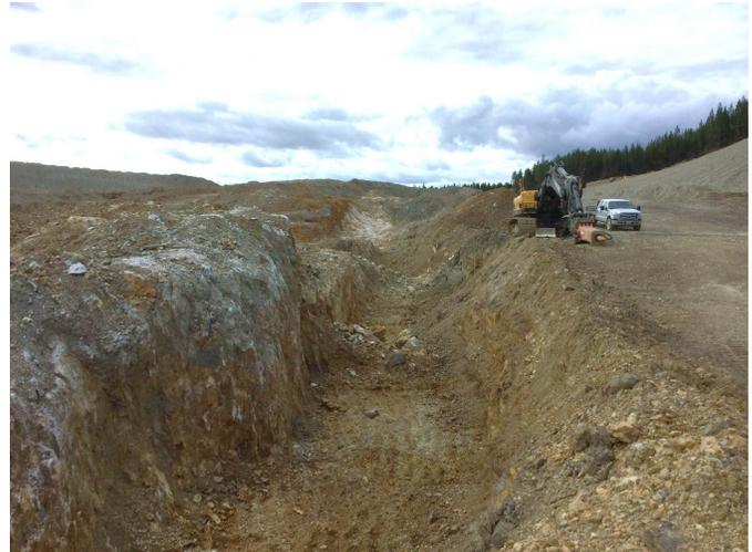
**Fig. 8.** First trenching in preparation to bench down and blast the Moose pit at Fireside mine.
