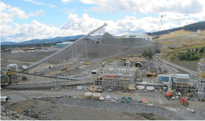
**Fig. 6.** Permanent secondary crusher under construction at Mt. Milligan mine. View is looking south.
