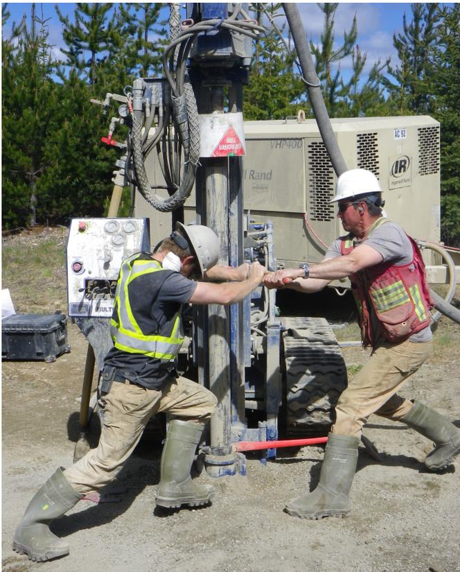
Fig. 11. Wildcat project, adding casing to reverse circulation drill rig.
