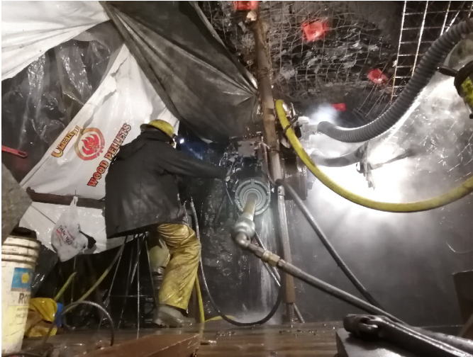
Fig. 6. Underground drilling at the Silvana project.
