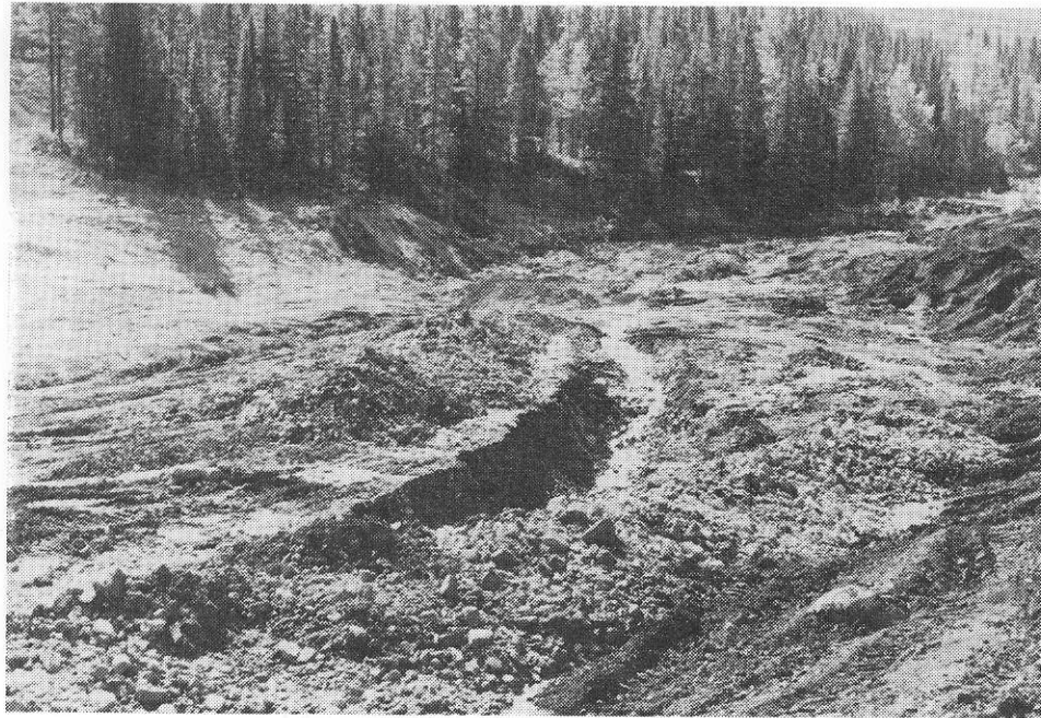
140 Excavation for rock drain collector along west slope of reservoir.
