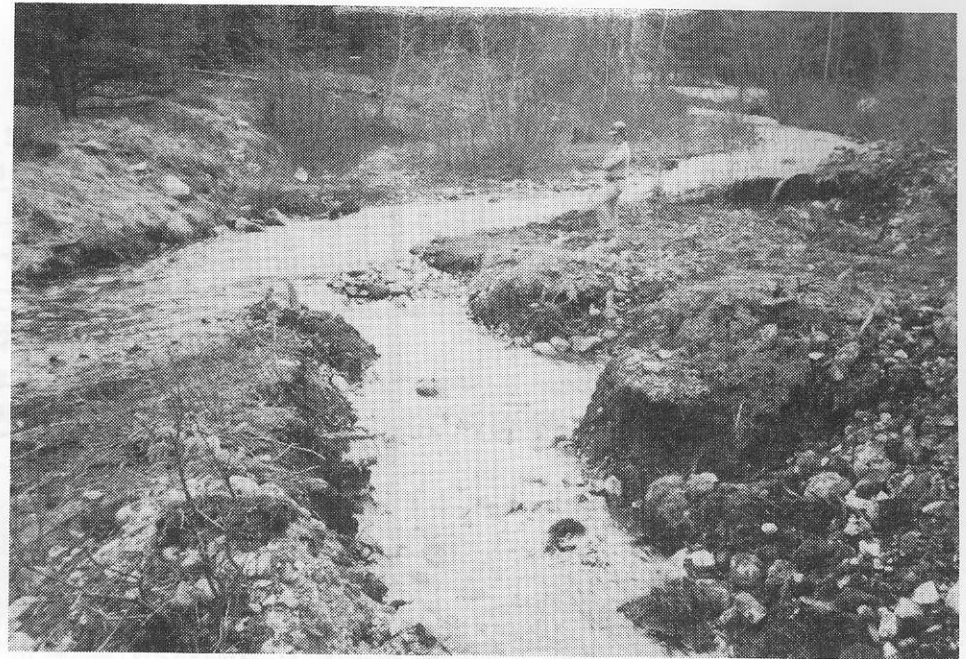
Corbin Creek flow being diverted along west side of reservoir (fork at bottom of photo). Flow was subsequently directed into rock drain.
