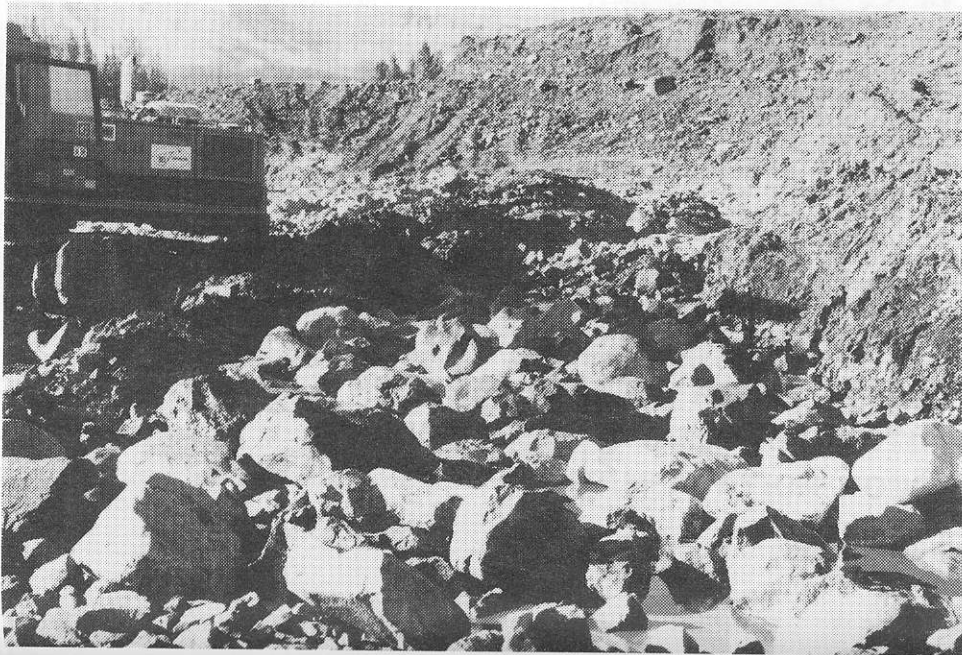
140 Excavation for rock drain collector along west slope of reservoir.
