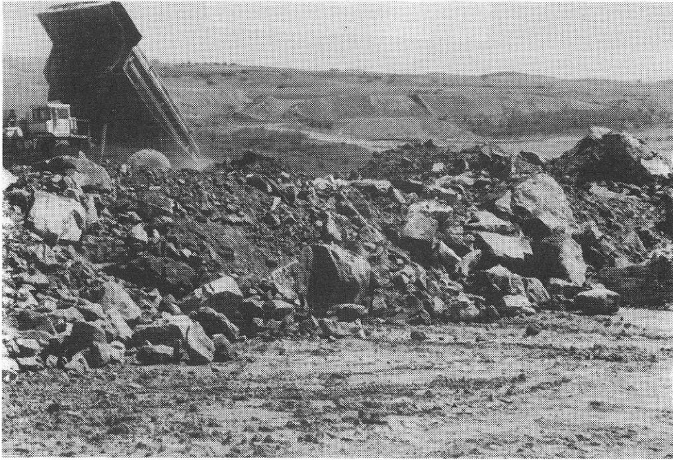
Picture No. 3 - Placing spoil lift. Lower area.
