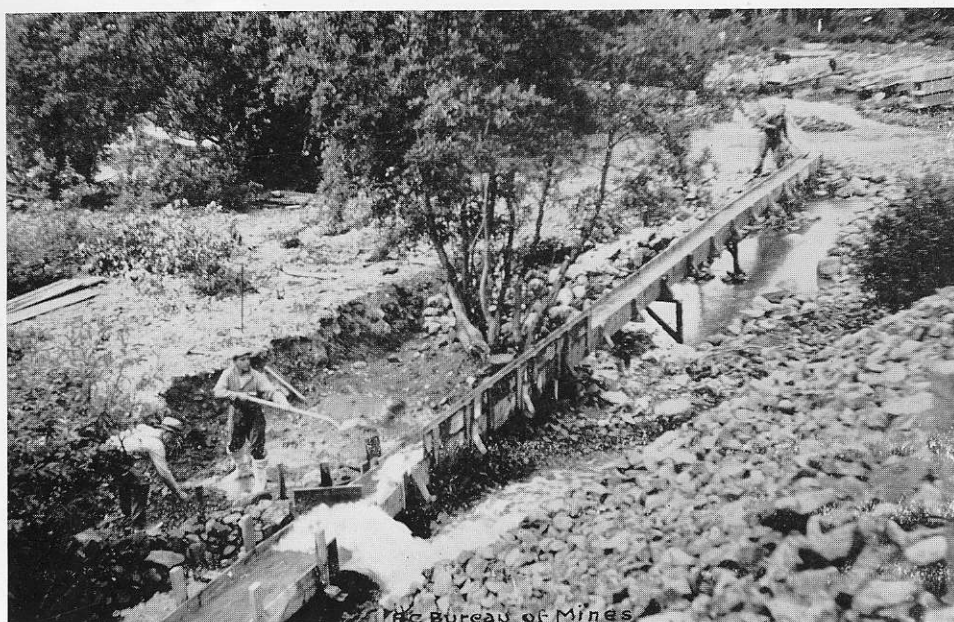
Spruce Creek, Atlin. Shovelling in to Sluice.
