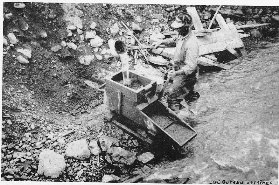
Spruce Creek, Atlin. Method of Washing Gravel with Rocker.
